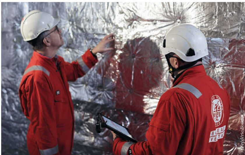
Insulation - inspection of pins distance for insulation material.
